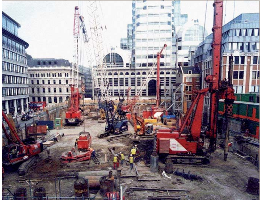
Fig. 5. Construction of a deep basement using the observational method
